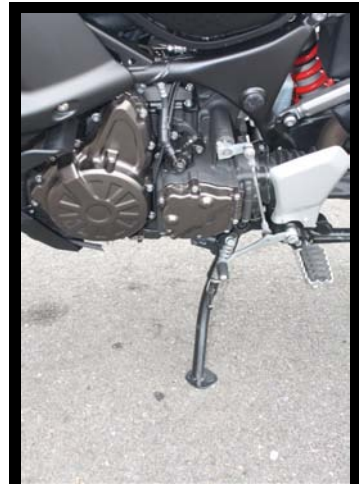
The kickstand, chassis, and all other metal parts should be checked for rust and corrosion
